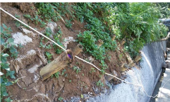
Gambar 4. Proses penetrasi material bambu
