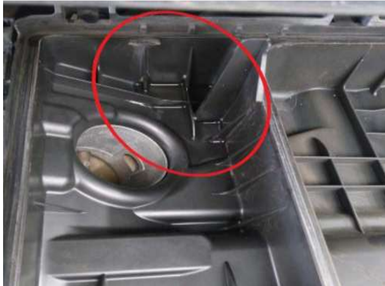
Figure 6 Gap in Air Filter (Source: 2018 research documentation)
