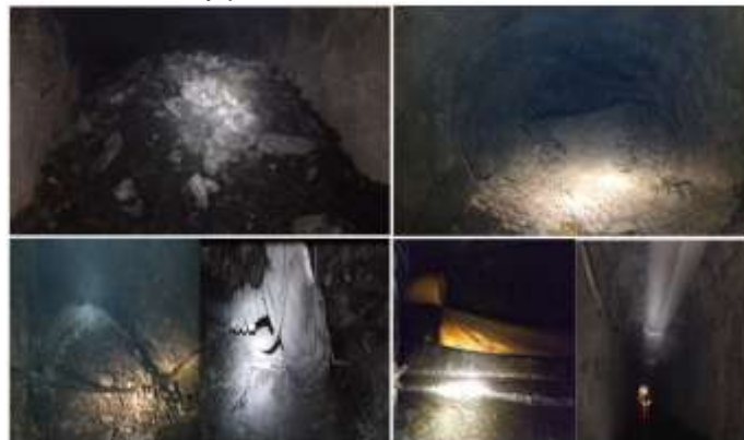
Figure 6. Muck after Blasting,services line top on stuck muck and broken down ventbag (Main Support Process)
