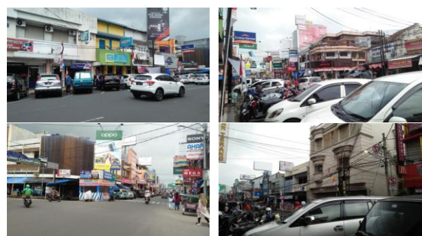
Gambar 6. Gambar Eksisting Ruas Jalan Segmen 3
