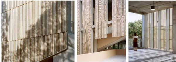
Gambar 17. Panel Perforated Alumunium, Gedung NUS School of Design & Environment 4, Singapore Sumber: https://nzeb.in/ & https://www.arch2o.com/
