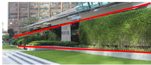
Gambar 10. Wind Catcher Gedung CIC Zero Carbon Park, Hongkong
