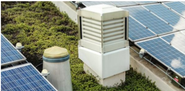
Gambar 9. Wind Catcher Gedung CIC Zero Carbon Park, Hongkong
