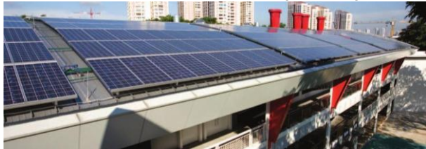
Gambar 2. Atap Solar PV berventilasi, Gedung BCA Academy, Singapore Sumber: https://www.hpbmagazine.org/
