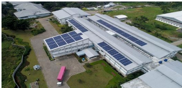
Gambar 3. Atap Solar PV, Gedung PT-Ungaran Sari Garments (PA6&7) Semarang, Indonesia Sumber: https://nzeb.in/
