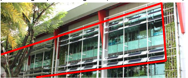
Gambar 14. Double-Skin Fasad Louvre terintegrasi panel Fotovoltaik, Gedung BCA Academy, Singapore Sumber: https://www.hpomagazine.org/
