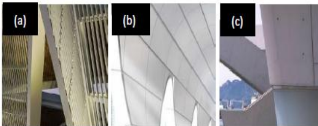
Gambar 10. Material bangunan (a) kisi-kisi aluminium (b) panel komposit aluminium (c) beton Sumber: www.archdaily.com
