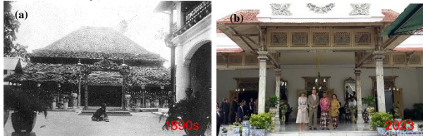
Figure 13. (a) Showing the boundaries and positions of the abdi raja (courtiers) who sit only in front of the building, (b) indicating the boundaries and positions between the Sultan and state guests at Gedhong Jene.
