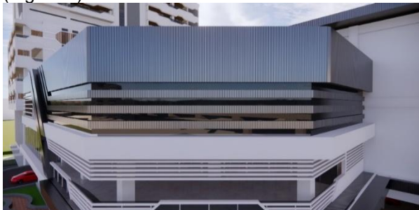
Figure 4. Aluminum Composite Panel Façade (Source: Author, 2023)
