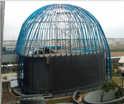
Figure 17. Hollow Aluminium Frames of Dome Construction.
