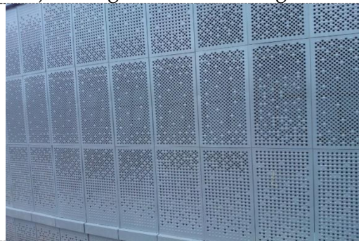
Figure 8. Perforated Aluminium Plate Secondary Skin.
