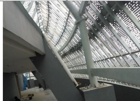
Figure 18. Main Structure of Dome Construction.
