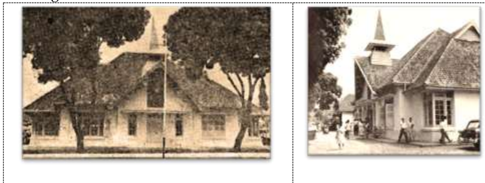
Figure 12. Façade Building of Wastukencana 40 Bandung (source: Southern Baptist Convention, 1955)
